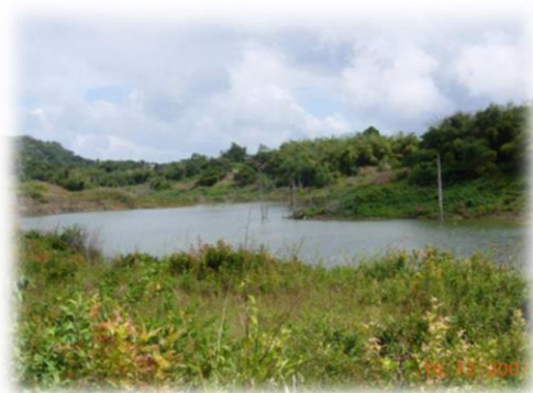
Figure 6-Settling pond at TCL
